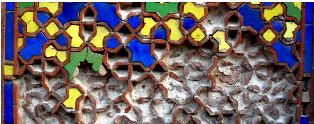
Figure 17: Loss of bond between the tile and the mortar
