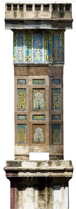
Figure 29: The southern face of the southeastern minar shows the detail of kashikari and exposed brick work
