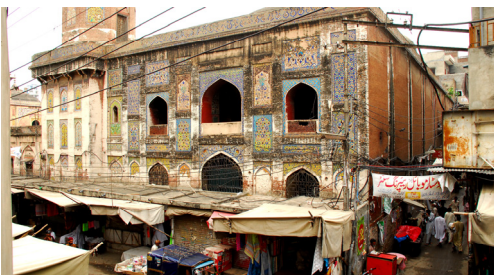
Figure 10: Northwestern corner of the mosque shows the level of commercial encroachments
