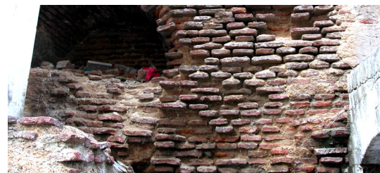
Figure 18: Sanding of mortar in brick masonry
