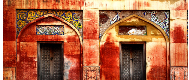
Figure 16: Fading of surface render (tazzakari) on the northern façade of hujra walls in the courtyard
