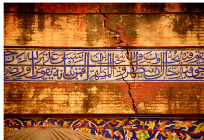
Figure 11: Major crack in the wall above the northern most archway of the prayer chamber
