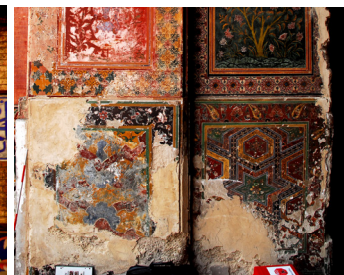
Figure 12: Rising damp in the main prayer chamber has damaged the fresco paint
