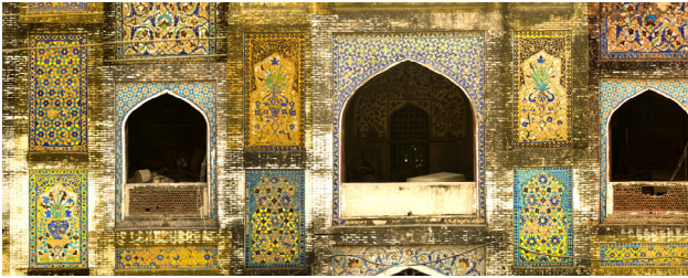
Figure 13: Deposits of soil and dust on the rendered and glazed surfaces of main prayer chamber facing north
