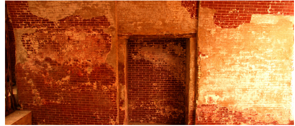
Figure 14: Efflorescence on the rendered surface (tazzakari) of the wall in the southern section of calligrapher's bazaar
