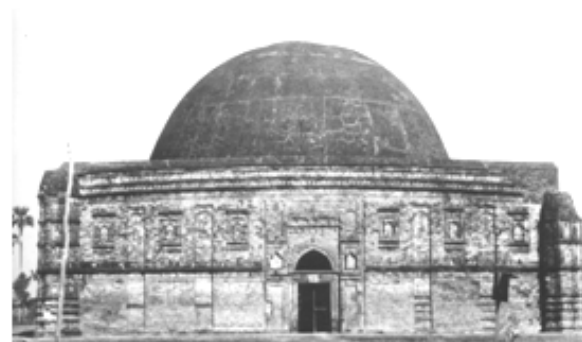
Figure 7: Eklakhi Tomb showing curved cornice
